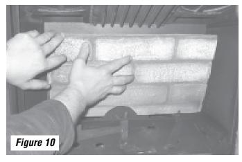
3. Install the left panel (B) bottom first and stand flush against left wall of firebox. Repeat for right panel (C) against the right wall of firebox.
